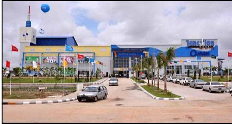
[Pic.9] Junction Nay Pyi Taw Shopping Mall
